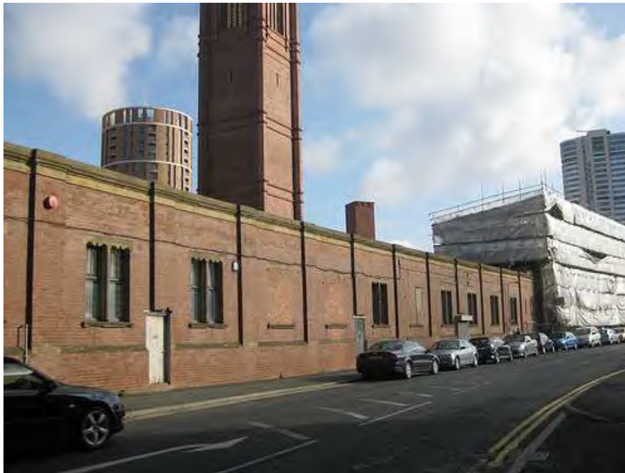
Tower Works, Globe Road, Holbeck, Leeds, LS11
