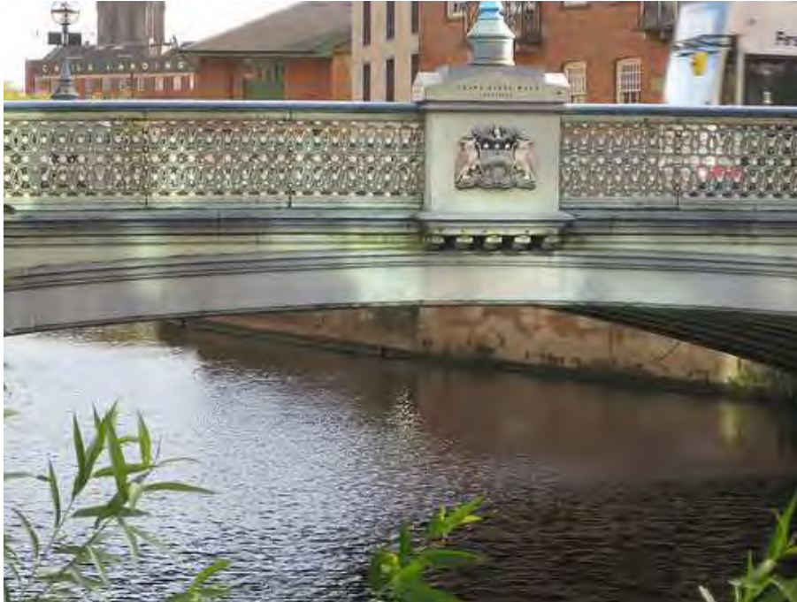
Bridge End, Leeds LS1
