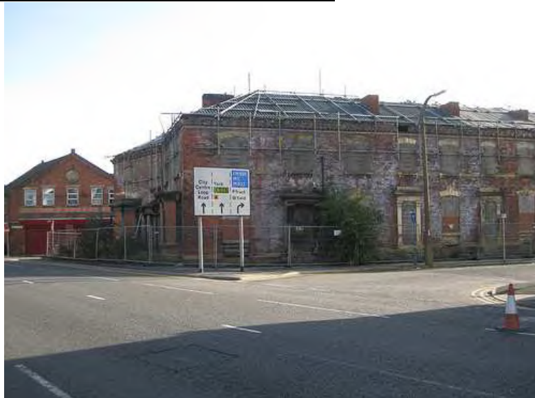
16 -18 Crown Point Road & 37-39 Hunslet Road, Leeds LS10
