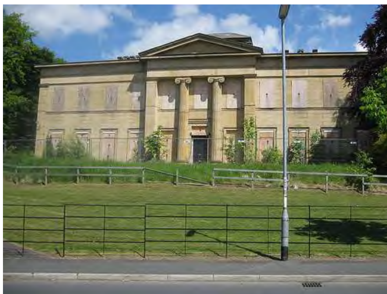
Harehills Lane, Chapel Allerton, Leeds LS7
